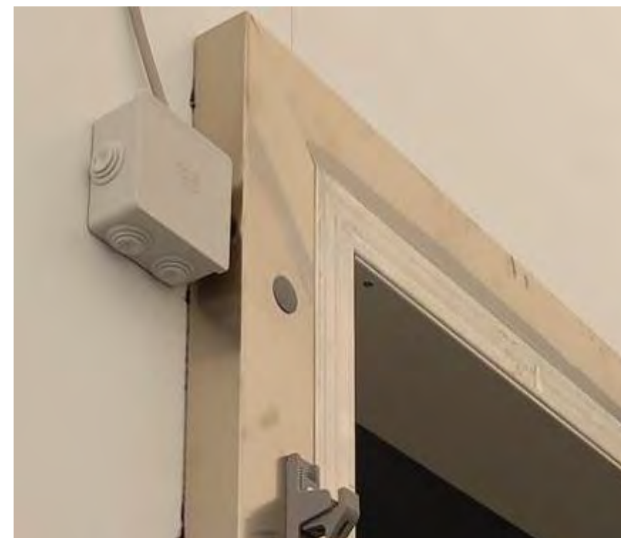
Frame with inox cover Gasket contact aluminium
