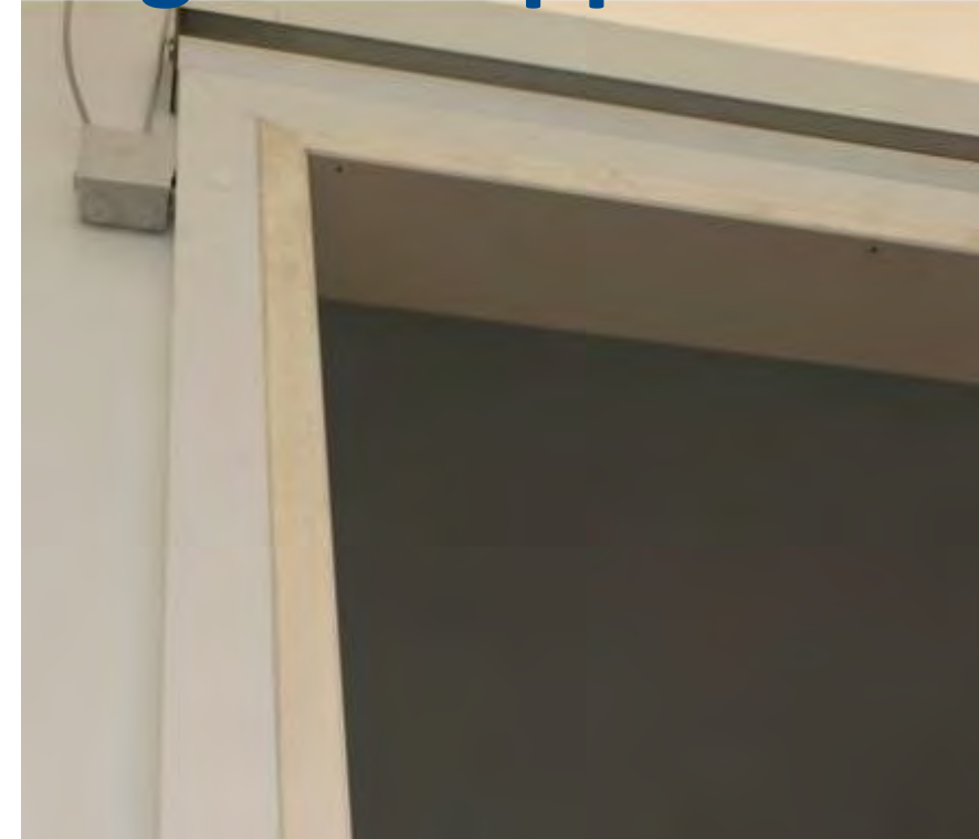
Frame PVC Gasket contact aluminium
